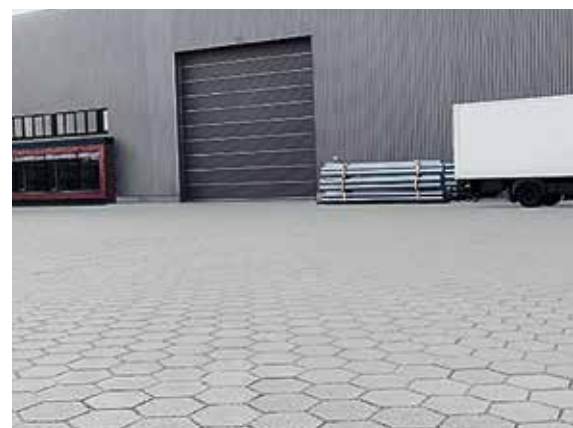
Abb. 27: GEOSTON carry protect, 12 cm Steindicke
